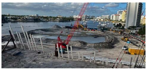
Batterpile installation with challenging geotechnical site conditions
