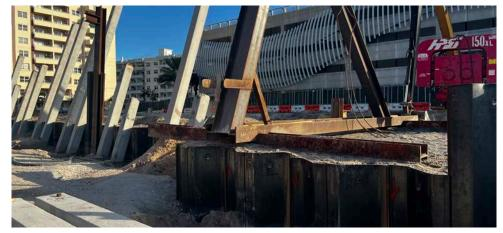
1,000 LF of sheetwall installation for new seawall in saltwater conditions
